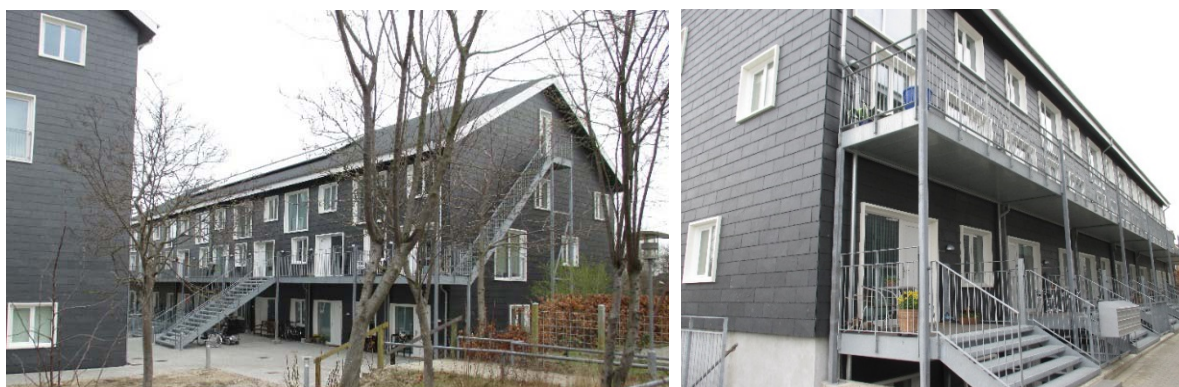
Figure 5. Sems Have after the renovation. The façade cladding is slate plates.
