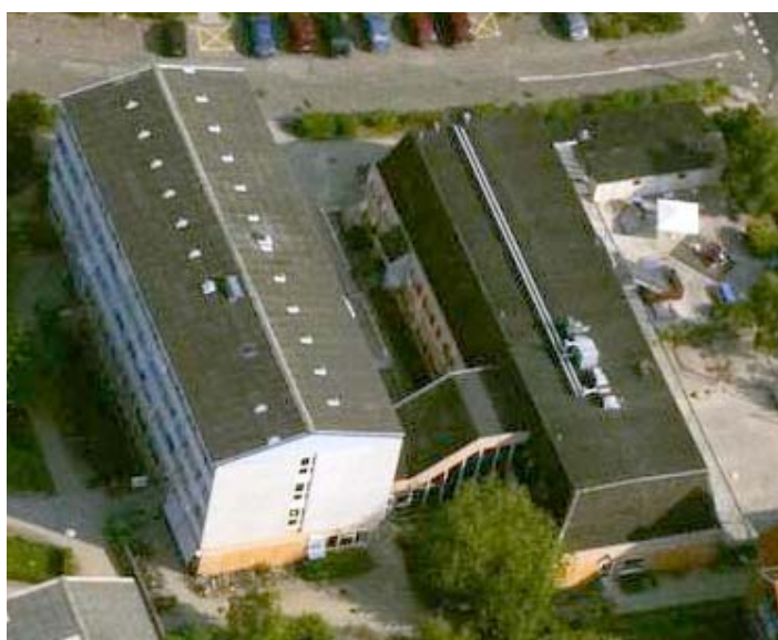
Figure 1. Sems Have before renovation.
