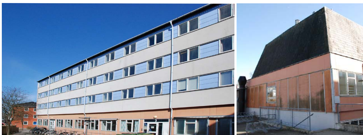
Figure 3. Block A (left) and block B (right) before renovation.
