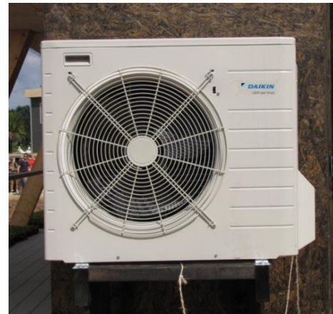
Figure 24 – Photograph of the Daikin heat pump installed on the wall of the technical room of EMBRACE
