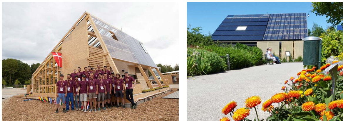
Figure 2. Photos of the EMBRACE house, during SDE2014 (left), and back in Denmark (right).
