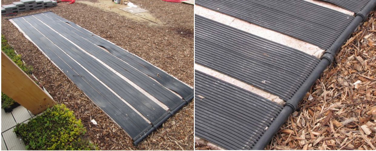
Figure 41. Photos of the unglazed collector in SDE2014.
