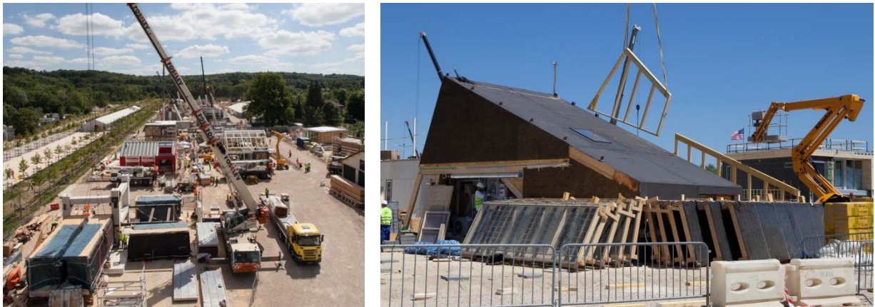
Figure 12. Cité du Soleil and EMBRACE under construction.
