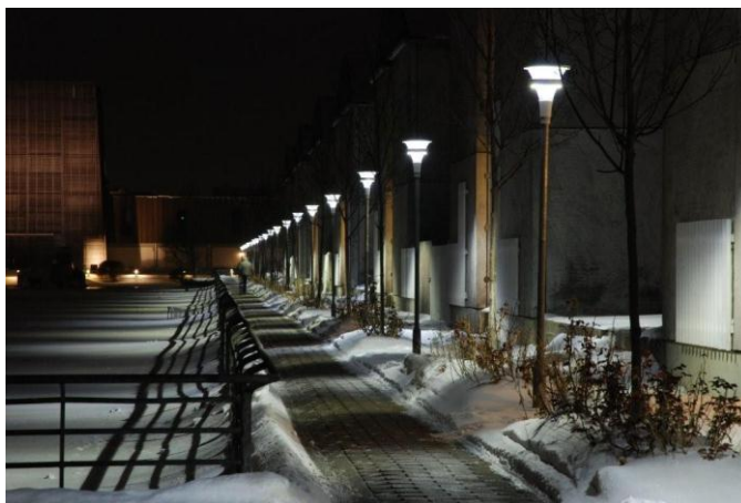
Figure 7: Albertslund street lighting (© City of Albertslund)
