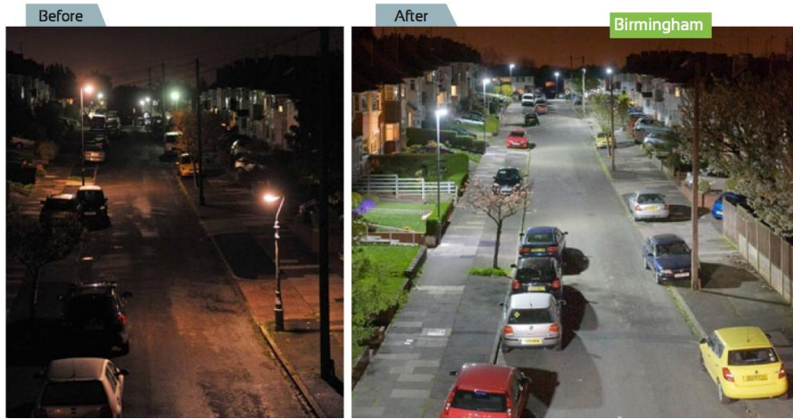
Figure 1: The impact of LED deployment in Birmingham (© City of Birmingham and Indal/WRTL)
