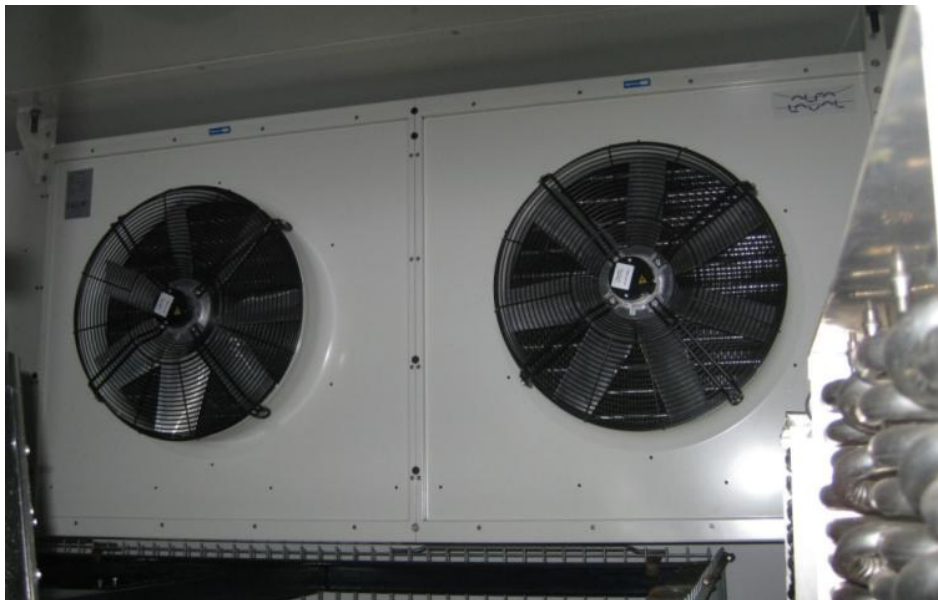
Figure 15: Air cooler mounted in climate chamber.
