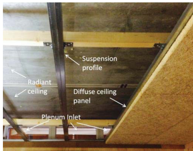
Fig.4. Diffuse ceiling panels and radiant ceiling
