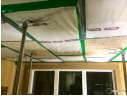
Fig. 6. Reduced diffuse ceiling area by covering vapor barrier.
