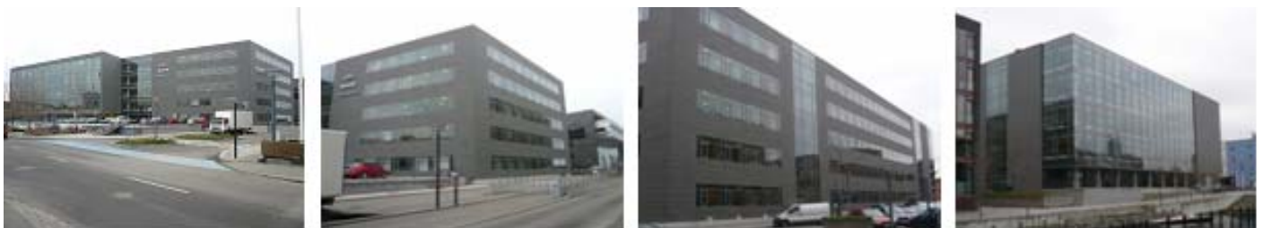
Figure 2: Facades of the building [1]
