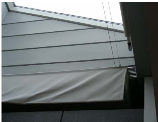
Figure 4: Convectors in the atrium area under the skylight [1]
