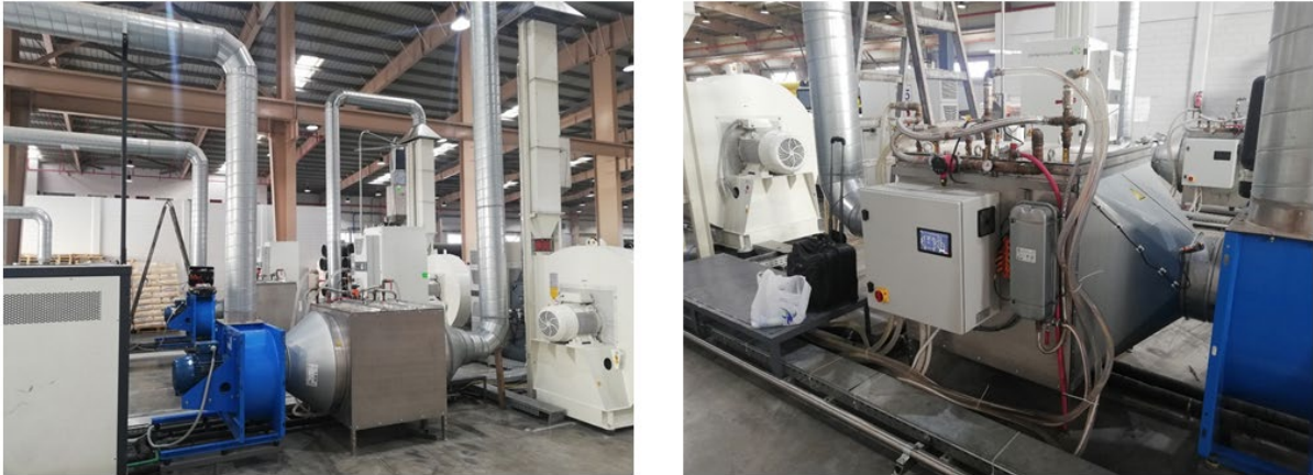
Figure 1.15: Labotek heat recovery unit installed in a production facility
