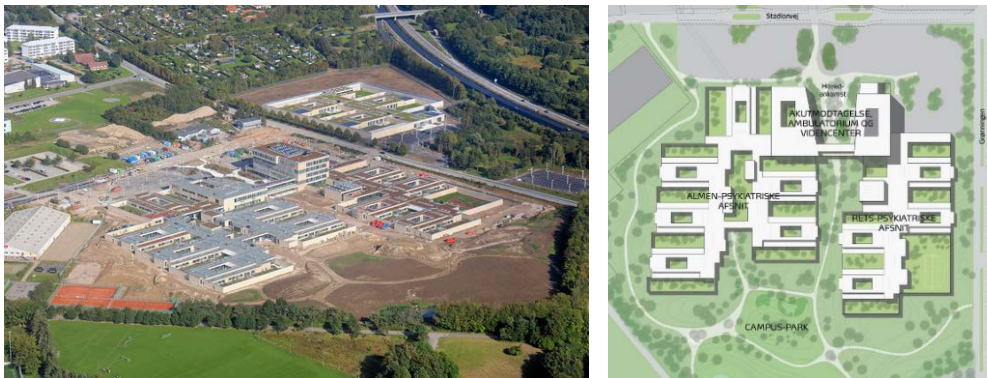
Figure 3-1: Aerial (left) and top (right) view of the Psychiatric Hospital
