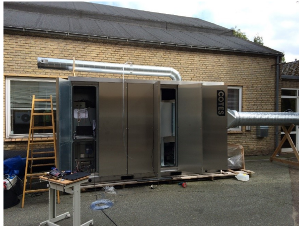
Figur 14: Foto af COTES DPC (Desiccant Dewpoint Cooler) unit
