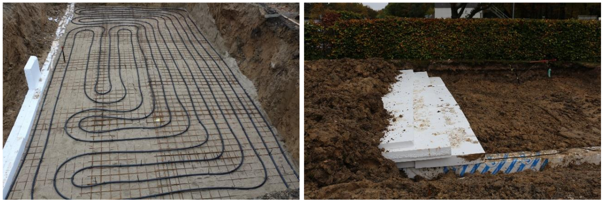
Figure 4. Pictures of ground storage during construction.
