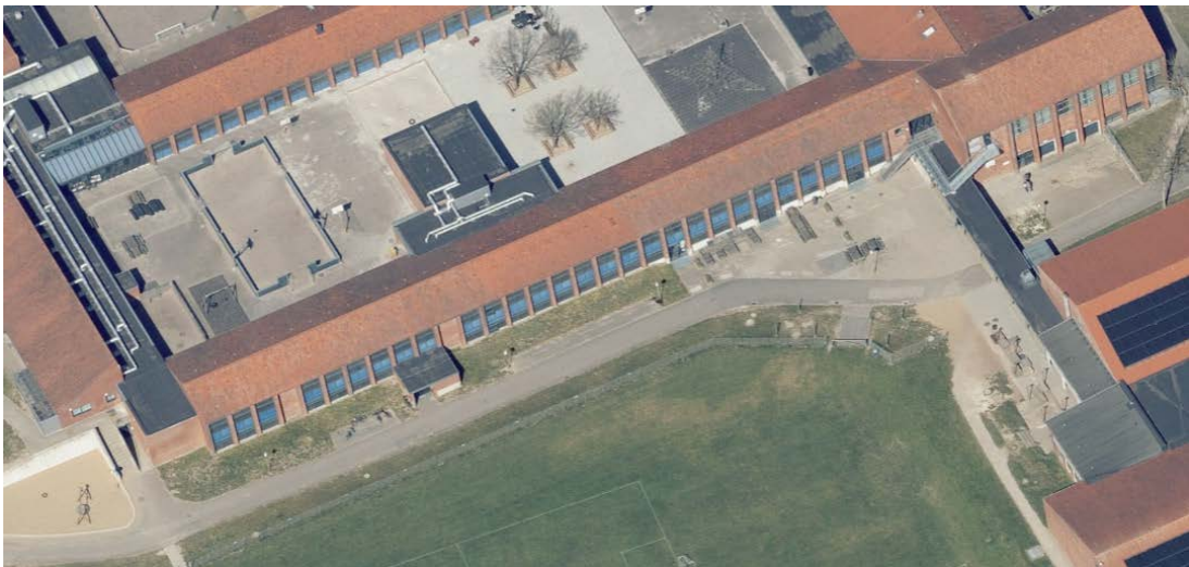
Figure 4. South-East facade of section D of the school.
