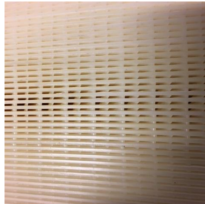
Figure 9 Parallel plate exchanger
