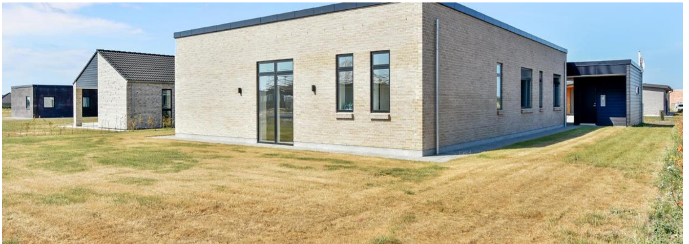
Figure 7. Residential house equipped by solar panels, heat pump and battery energy storage which is located in Ikast, Denmark.
